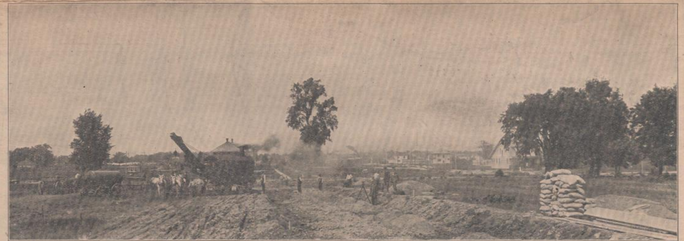
Harrison Hill in the Making—The Steam Shovel at Work on Harrison Blvd.
